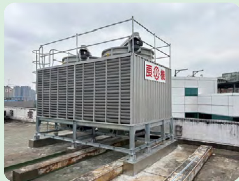
Replacement of cooling towers (Linkou Headquarters)
