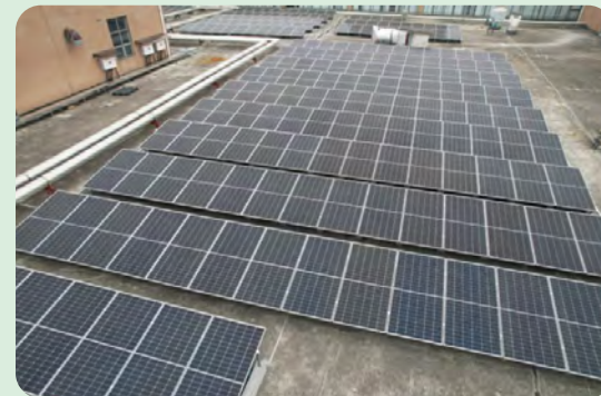
Installation of Solar photovoltaic (PV) system at Pihong (Dongguan)
